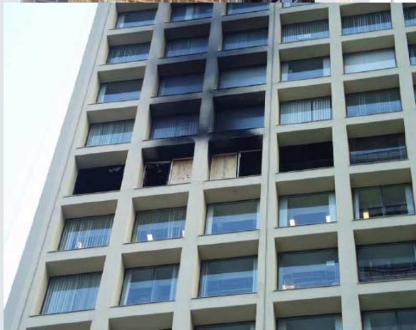
Figure 5. View of north side of the Cook County Administration Building
