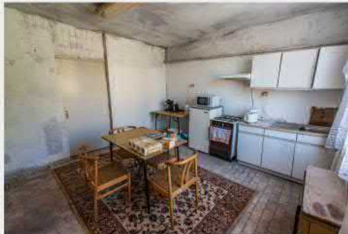
Site preparation, construction
