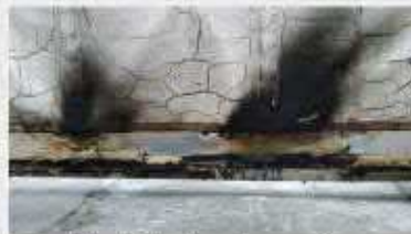
Fig 13. Test specimen, after the test
