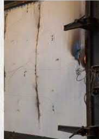
Fig. 8. Horizontal deformation of the wall, during the test
