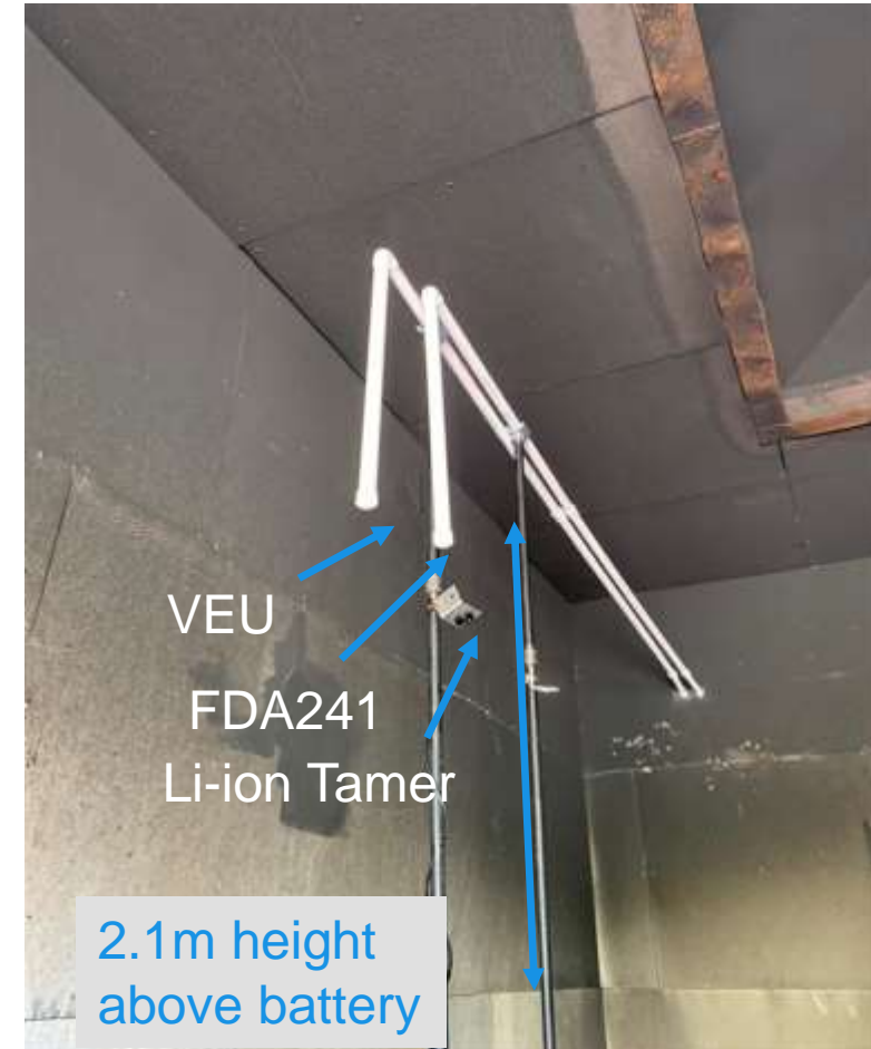
Setup B: Battery abuse by Over-Charging
