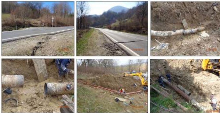
Figure 6. Gas pipelines affected by landslides – area 1
