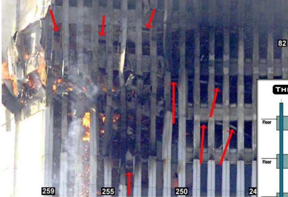
Figure 9-79. This photograph is a blow-up of a portion of the photograph shown in Figure 9-78. It shows the north face of WTC 2 and includes window 80-256 and the cold spot. The intensity levels of the original have been adjusted, and column floor numbers have been added. Arrows highlight hanging objects visible through windows on the 79th, 80th, 81st, and 82nd floors.
