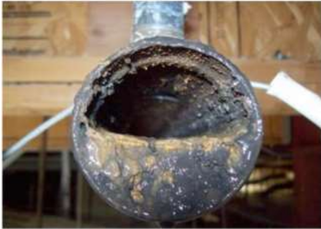
50% Blockage (California, 5 year old system )
