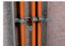
Fastening with threaded rods and side nuts in the range
