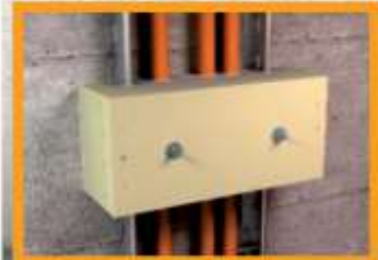
Function maintenance – standard support structures, vertical ladders, strain relief
