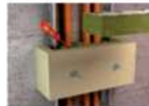
Mineral wool filling for flexible cable assignment
