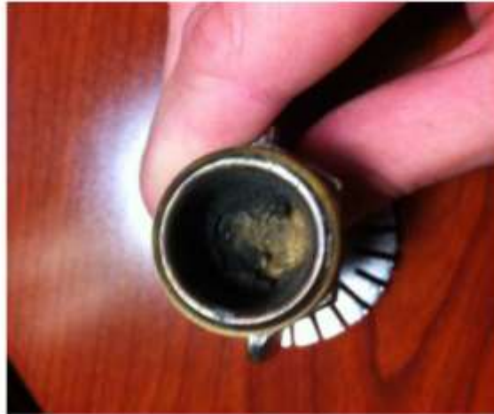
Failed Sprinkler Head (Illinois, 12 year old system )
